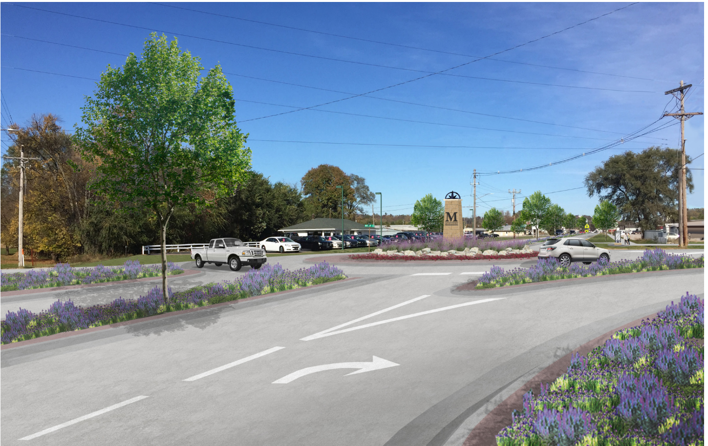
Figure 19: Design concept for focus site two. The perspective shows a roundabout style intersection with landscape medians, street trees, a paver splash pad, designated right-turn lane onto Sampson Street, and monument signage/sculpture at the center of the roundabout.
