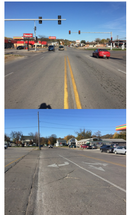
Figure 10: Existing conditions photos of focus site four.
