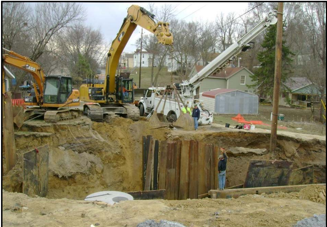
West Hill Sewer Separation Project
