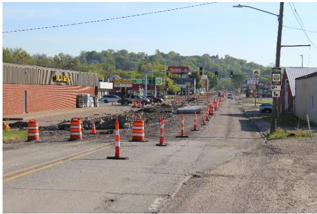
Pavement removal has been completed in the southbound lanes with sanitary and storm sewer work underway. Reconstruction of the southbound lanes will begin once the underground work has been completed starting near the Pearl Street intersection.
