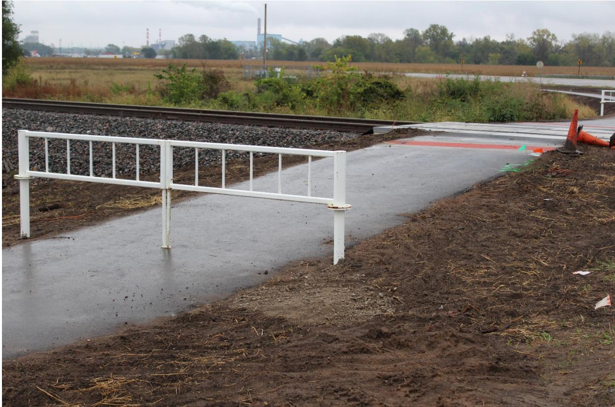
**GATES WERE** installed where the Kent Stein to Deep Lakes Park trail crosses the Canadian Pacific tracks on Dick Drake Way. The gates are a safety measure in addition to the crossing arms, lights, and sounds to prevent pedestrians and bicyclists from crossing the tracks when trains are present.
